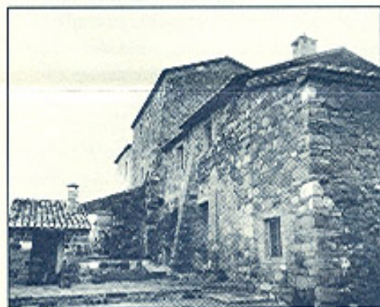
One of the ancient buildings at Trinoro restored by Andrea Franchetti.
